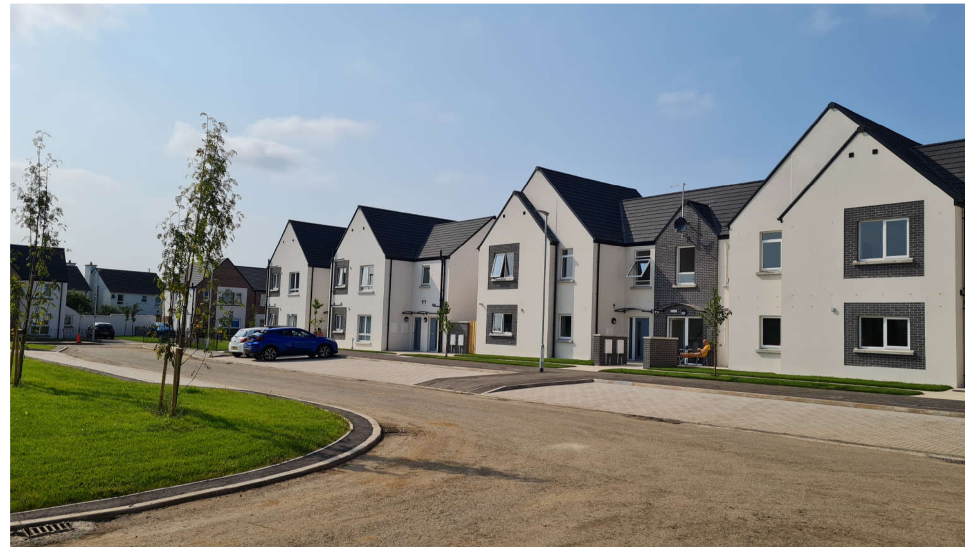
Typical Example of Dual Frontage Apartments at Sites 77-82
